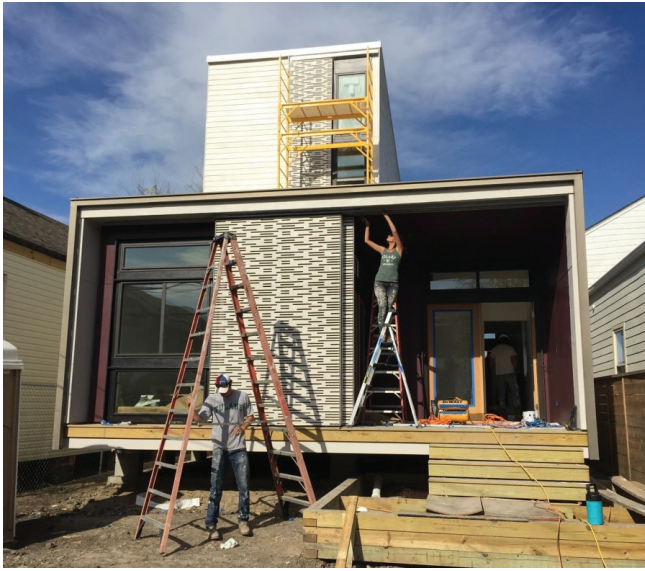
Figure 3. URBANbuild 11, front construction.
